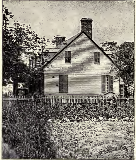
THE WEST HOUSE AT YORKTOWN (Showing the shot holes)
